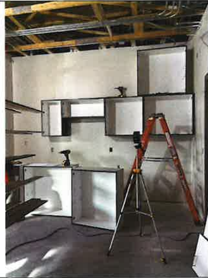
Meeting room casework being installed.
