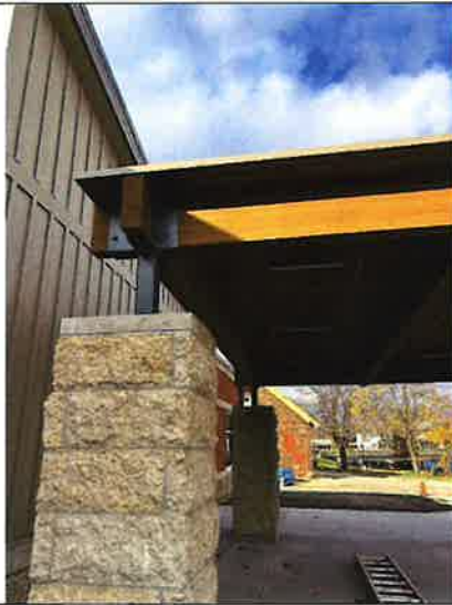
View of painted steel at shade structure.
