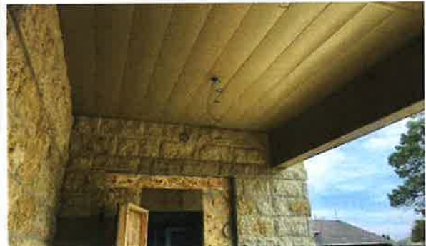
View of the front entrance with the installed metal soffit panel.
