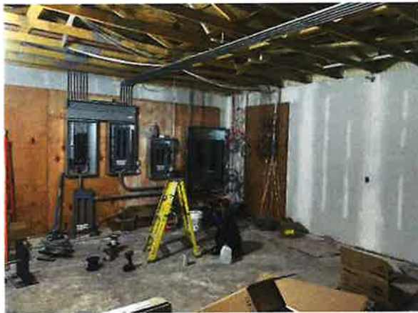
View of Mechanical 108 and work in the NW corner.
