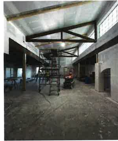
View in the clerestory, looking east towards the fireplace. The translucent panel and wall finish are in place.
