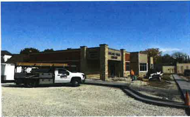
View of the main entrance.
