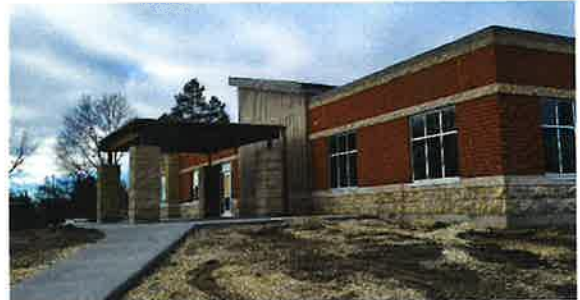
View of the exterior from the north of the site, looking south at the patio slab.
