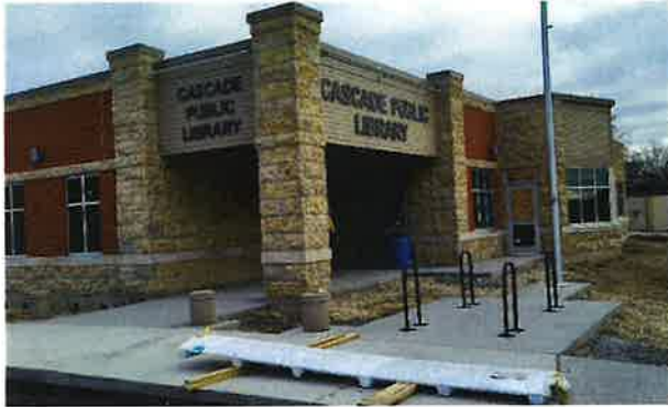
View of the main entrance.
