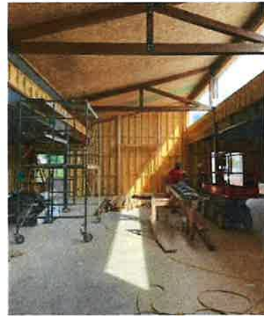
View in the clerestory, looking east towards the fireplace.
