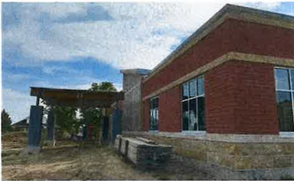
View of the east wall and shade structure, looking south.
