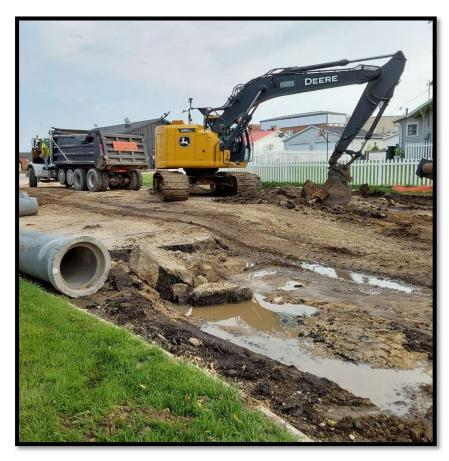
Wednesday the crew spent the day removing the remaining old storm sewer pipe and structures from the entirety of the project. This amounted to over 800 feet of storm sewer and 10 structures removed.
