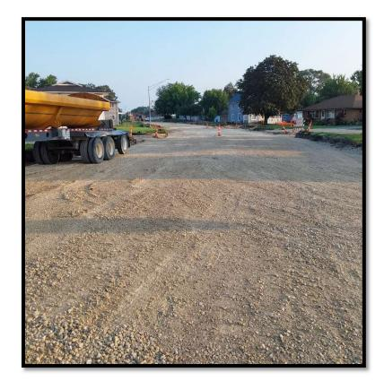
Thursday the grading crew continued pavement removal and coreout on the rural portion of the project, removing about another 250 feet of material as well as starting to dig in subdrain on that stretch..
