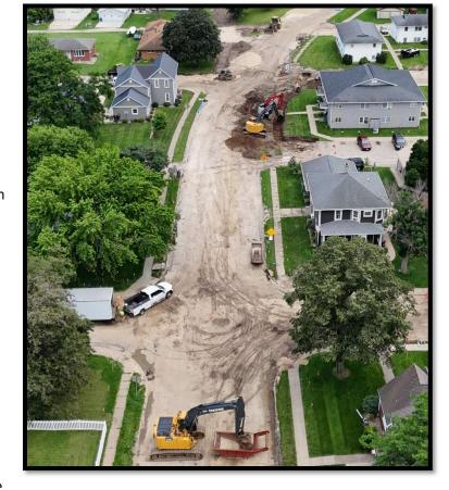
Thursday the crew continued storm sewer installation to the north along the east curbline of IA 136/Johnson St. They installed about 170 feet of concrete storm sewer pipe while also excavating where new storm drainage structures will be located.
