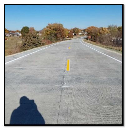
roadway. Due to DOT smoothness requirements, portions of the roadway still need to be diamond ground to meet specifications. This work cannot be completed for multiple weeks due to grinding contractors being booked up until then. The grinding work will at that time be done under lane closures with flaggers, allowing traffic to still use the roadway while the work is being done.
