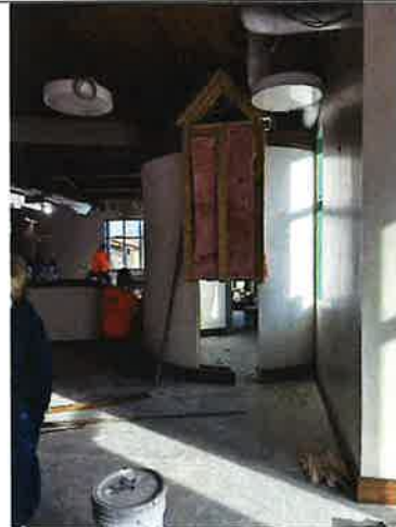
Silo in Children's collection, Trim being installed.
