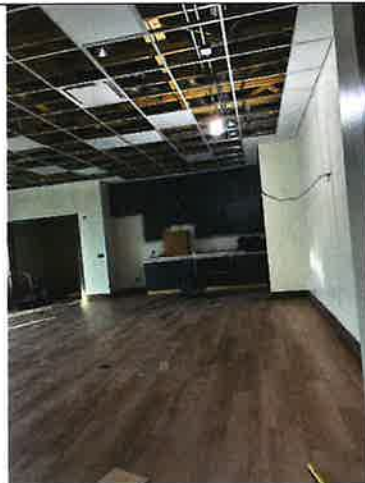
LVT being installed in Meeting Room.
