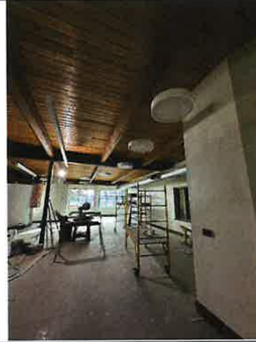
View from Children's entrance toward the Silo.
